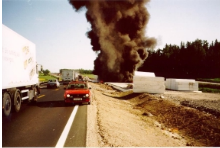
Figure 1. Fire causing total loss of non-flame-retardant EPS-block geofoam being used as lightweight fill on a road project (Euroroad E6 in Vestby, Norway). This is one of only two known projects in the world where there was a total loss of EPS-block geofoam due to fire. The loss in each case was due to contractor error (courtesy of Mr. Tor Erik Frydenlund of the Norwegian Road Research Laboratory).
