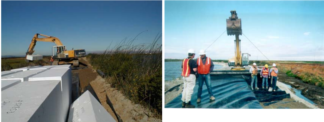
(a) (b) FIG. 2. Roaring River Slough project under construction.
