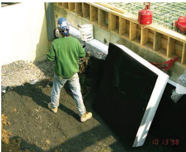
Figure 3. Geofabric Compressible Inclusion Used on a Bridge Project in the U.S.A
