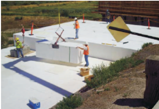
Figure 1. EPS Blocks Used for Road-Widening Project on Soft Ground in U.S.A
